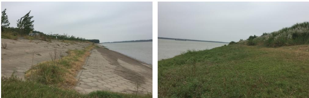
(a)水泥护坡 (b)钢丝网格护坡
